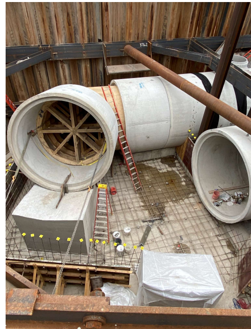
Figure 3 - Installation of the first inclined section of RCP. Photo Credit: Chad Koglin
