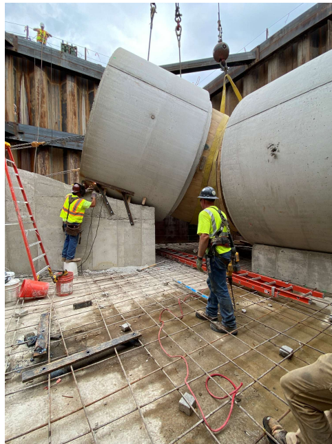
Figure 2 - Workers secure and inclined section of RCP. Photo Credit: Chad Koglin
